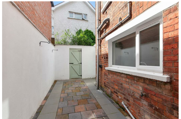
South facing paved courtyard garden to rear, plumbed for washer / dryer.
