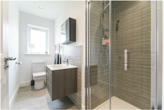
White suite comprising of corner shower cubicle with stainless steel taps and tiled walls, low flush w.c and square sink basin with stainless steel mixer taps with tile splashback and vanity below. Tiled flooring and recessed spotlights.
